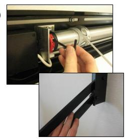
**13.** Replace the motor cover and make a final operational check of the mount. Installation is now complete.
